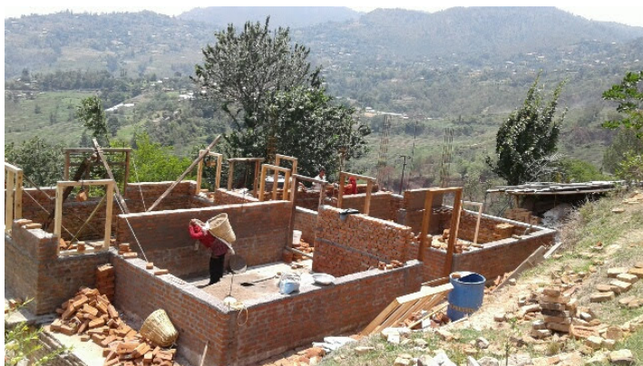
New home building in post earthquake Nepal
